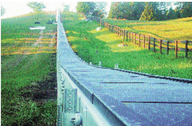
Mansfield Ski Club in Ontario installed the longest Magic Carpet last summer—a whopping 800 feet. The Carpet will move 1,500 people per hour at full capacity.
