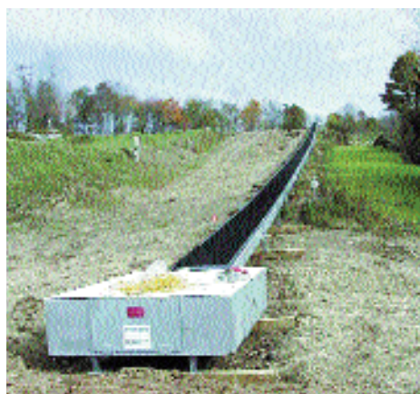
A Magic Carpet installation at Woodbury Ski Area, Ct.
