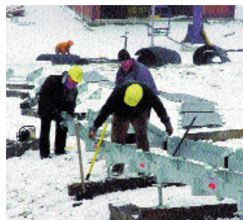
Star Lifts' SunKid being installed at Smugglers' Notch.
