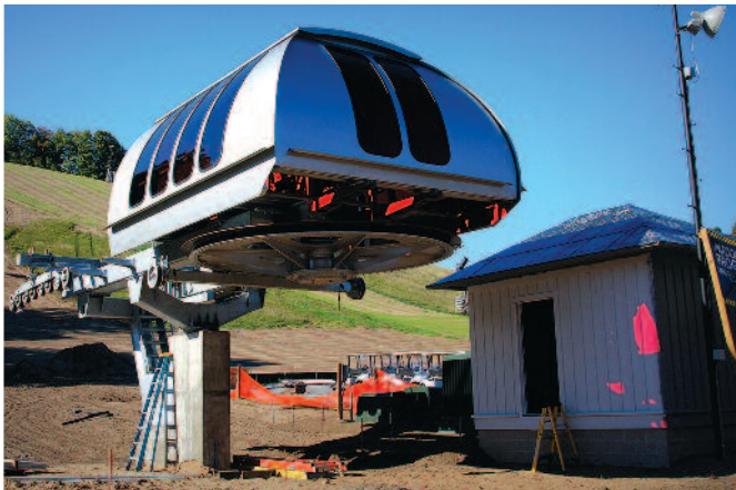
TOP ROW: Left: A terminal is installed for Lutsen Mountain's new detachable 6-pack from Leitner-Poma, which covers almost 3,600 feet. Right: Breckenridge installed two Leitner-Poma lifts—a detachable 6-pack and a fixed-grip quad. Shown here is the lower end of the fixed-grip quad. SECOND ROW: Both pictures are of Doppelmayr's detachable quad installed at Snowbird, Utah, which will carry 1,800 people per hour this winter. THIRD ROW: Left. These two conveyors by Star Lifts were installed in the beginner area at Brian Head, Utah, which is under new ownership. Right. This 410-foot conveyor from Magic Carpet was installed at Fernwood Resort in Pennsylvania. BOTTOM ROW: Crystal Mountain, Mich., is the proud new owner of this fixed grip quad from SkyTrac.
